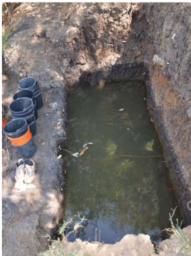
Figure 17: Water in Area E.
