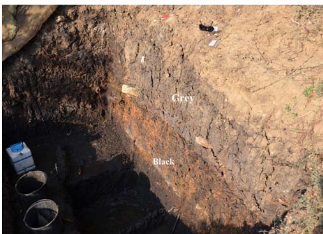
Figure 16: Contact between upper grey and lower black mud at eastern section of Area E. Lower dark mud is oxidized after exposure to air.
